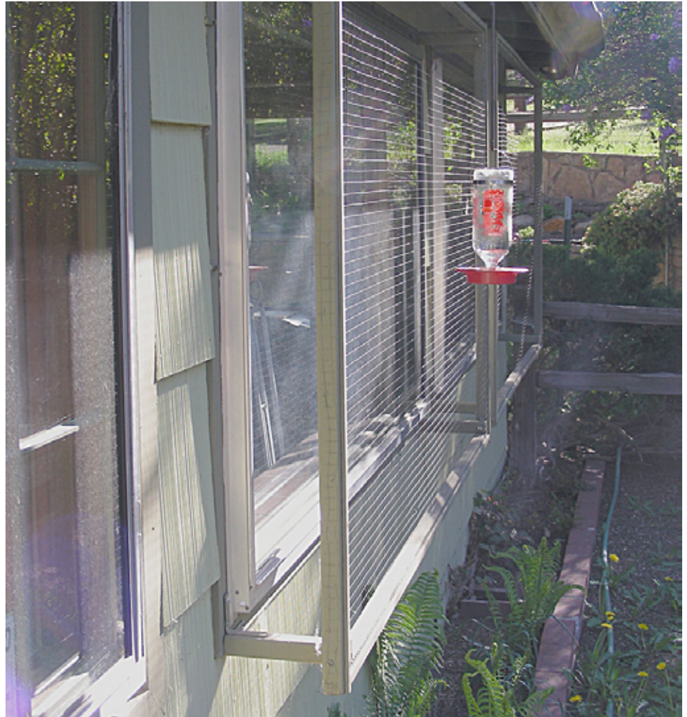
Side view of screen mesh stretched tightly over metal frame.
