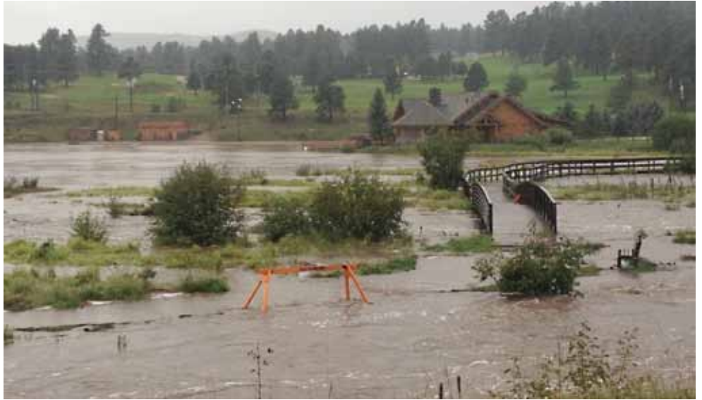
Flood waters inundated the area around Evergreen Lake House on Sept. 13. Photo courtesy of JustAroundHere.com, photographer unknown
